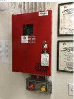
a. When a single sensor detects smoke (or dust) in the air, it will sound a very loud warning **BELL** alarm, which is in the equipment room. When that sounds, someone needs to check the equipment rooms. Be sure to take note of which sensor is showing the red LED light before resetting the system. This will assist in narrowing down a possible faulty detector if there is no visible smoke.
